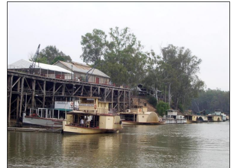
What remains of Australia's inland maritime history rests at Echuca on the Murray River. The wharf is very high to cope with varying river level.
